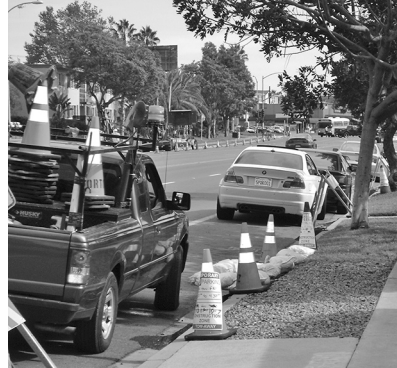
Crews work to ensure water reliability along Clairemont Drive.
